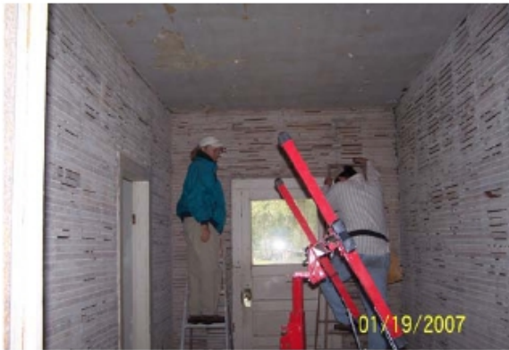
David & Marilyn Webb working on the 100+ year old Lafite House
